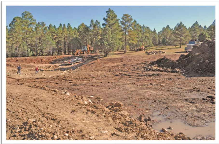
The pond cavity half excavated. Note the pile of rocks and large pile of reserved topsoil to the right of photo. (2010 Photo by J. Riddick)
