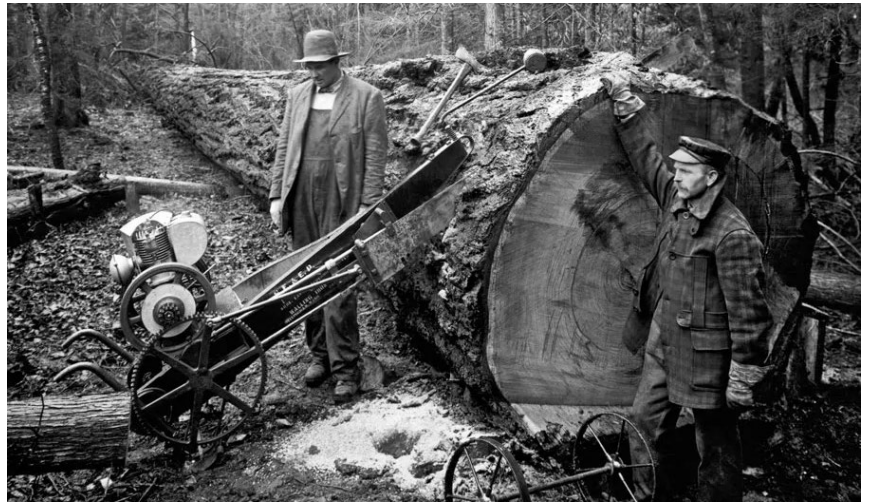
A motorized and portable drag saw being used by lumbermen in Washington, Bellingham, Washington, circa 1916. Photo credit: Getty images
